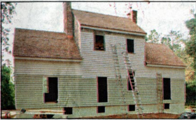
The restoration of Cabaniss House has progressed quite well.
